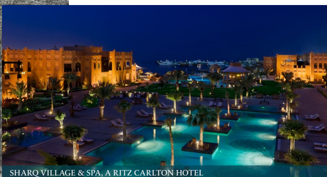
SHARQ VILLAGE & SPA, A RITZ CARLTON HOTEL
